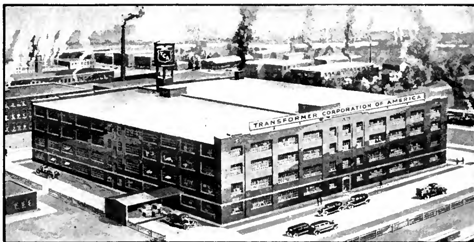
The Transformer Corporation of America has removed to the new plant pictured above. Their new equipment will have eight times the capacity of the former factory.
